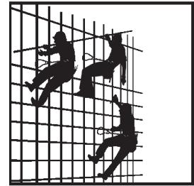
**Climbing rebar** – Workers are permitted to free-climb concrete forms and rebar to reach work areas. The maximum free-climbing height is 24 feet. The horizontal bars must be spaced not less than six inches, or more than 16 inches on center. When rebar spacing is more than 16 inches on center, use a ladder or lift to reach work areas. Upon reaching a work area, you must use a personal fall-arrest system, safety net, or positioning-device system for fall protection.
